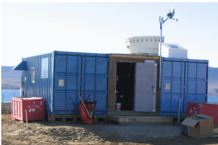
Figure 11: Two sea containers were insulated and equipped in Toronto and airlifted to Eureka by a C-130 Hercules. They are situated near sea level at the site of the Eureka weather station.
