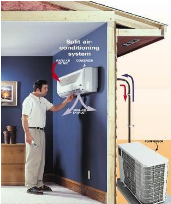
Split air-conditioning: Wall mounted indoor unit and outdoor unit
