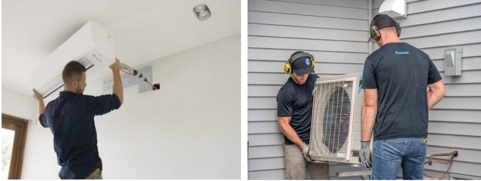
installation, requiring refrigerant piping connections on site
