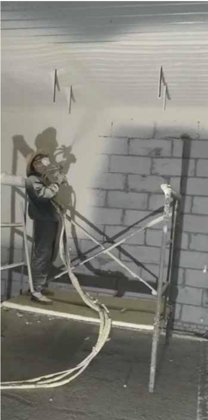
Dacheng Wan Fu Chemical Co. Ltd spraying foam in a cold storage warehouse in Hebei Province, China.
