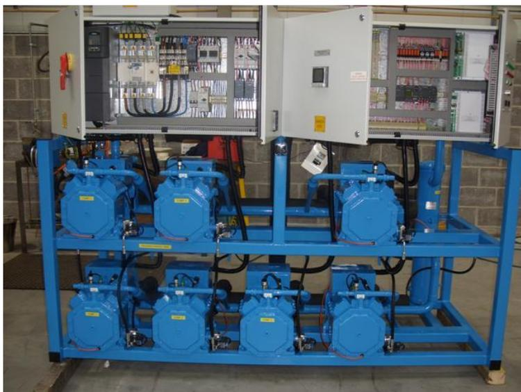
Factory built stand-alone systems have a small refrigerant charge and low leakage rates.
