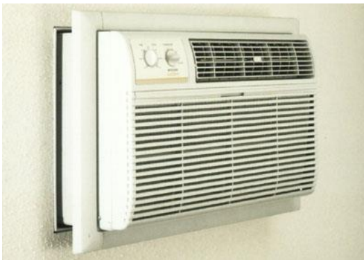
Through-the-wall air-conditioning unit
